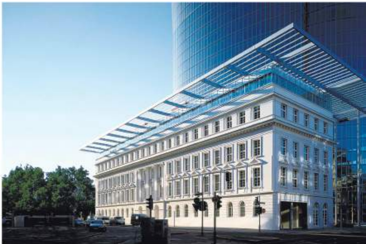
GAP 15 office building, Düsseldorf, Germany
